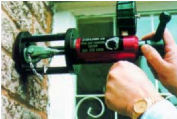
Testing Ring Anchors
